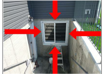
Exterior trims/casing around the egress window are not installed.
