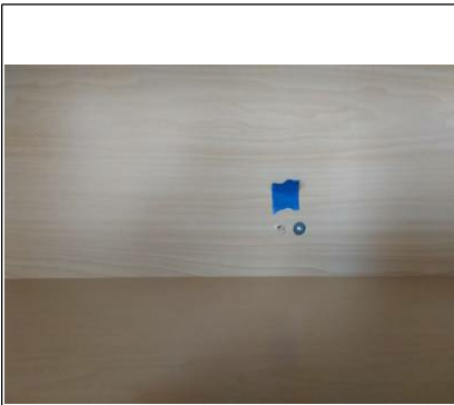
Extra hole punched for wall cabinet.
