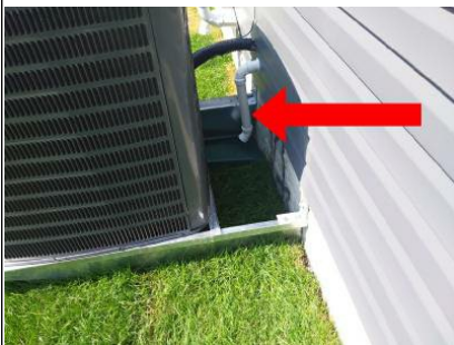
Sump pump discharge is terminating below grade behind the air handler. Recommend adding an extension to get water away from the house. Check for proper pitch. The alternative is to move the position of the discharge line.
