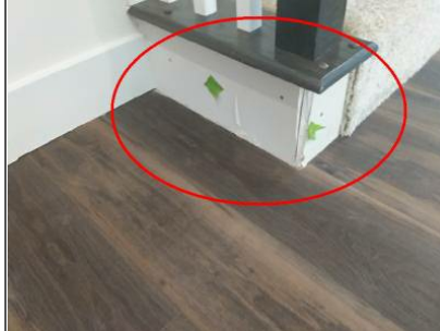
Bottom of landing in foyer is incomplete.
