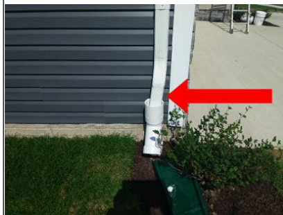
Front left downspout is not plumb.
