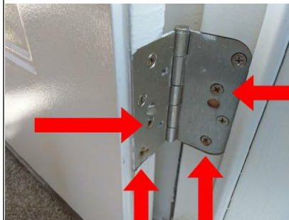
Screws are rusting on bottom hinge of egress door.
