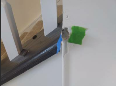
Incomplete drywall at top of bottom rail to upper level.
