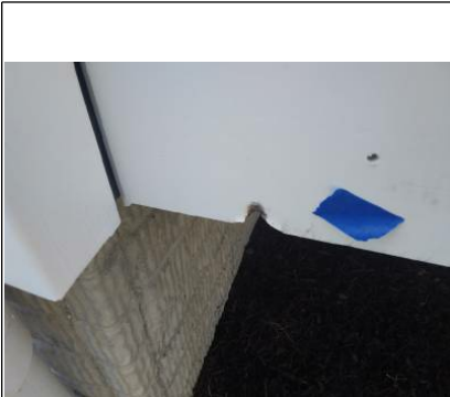
Gouge out of fascia board close to the house on the left side.
