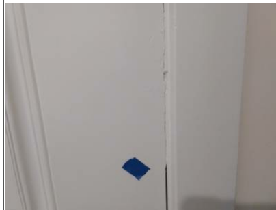
Sloppy finish on hinge side of front door.
