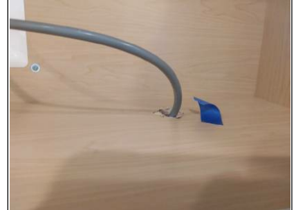
Cabinet penetration above the microwave should be sealed.
