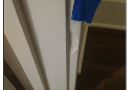
Casing next to bottom hinge on left door of coat closet is damaged and poorly repaired.
