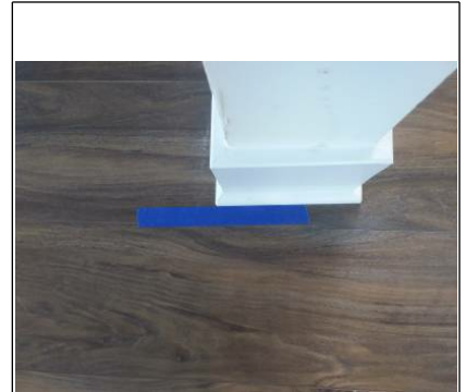
End of wall on left side of dining room opening is out of square.
