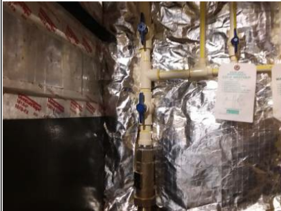
Main water shut off is not clearly marked.
