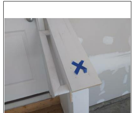
Top right plate on staircase is loose.
