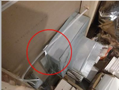
Return is not properly set to the wall.
