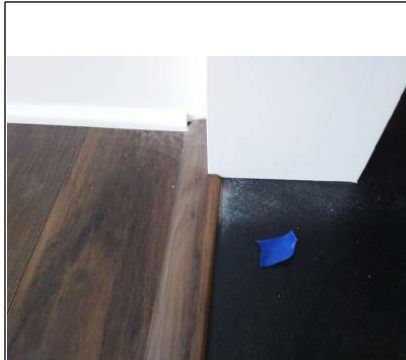
Paint over spray on left side of fireplace hearth.
