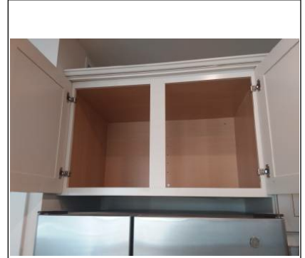
Shelf is missing in cabinet over the refrigerator.
