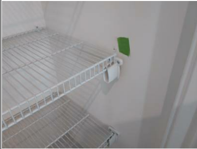
Shelf bracket not properly installed in pantry.
