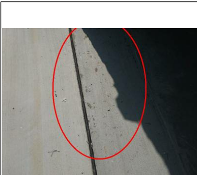
Gap between drywall and casing on the left of the fire door.
