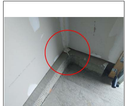
Top right plate on staircase is loose.
