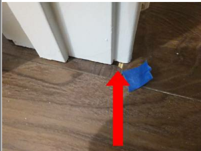
Flooring is cut short on inside of coat closet at the bottom of the left side of the door casing.
