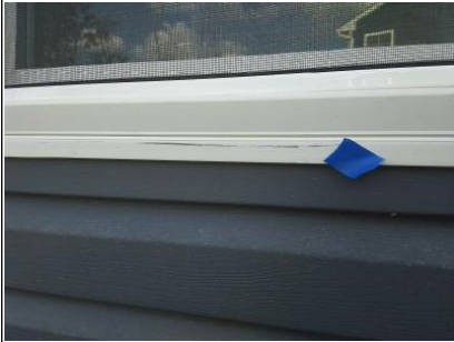
Molding is scratched under right side double windows.
