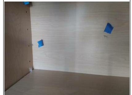
Sharp ends of nails sticking through back of base cabinet for island closest to the family room.
