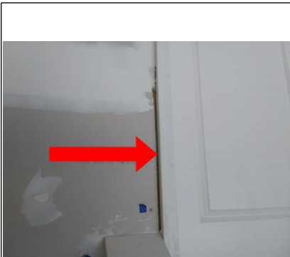
Gap between drywall and casing on the left of the fire door.
