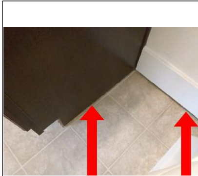
Shoe mold is missing around the vanity and and the base mold.
