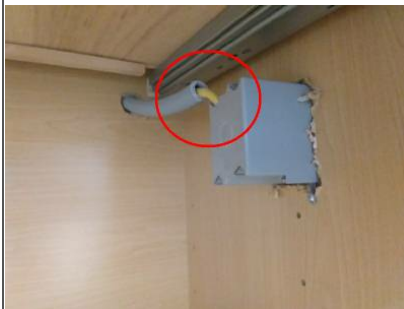
Gap between conduit and Junction Box on the end of the peninsula.
