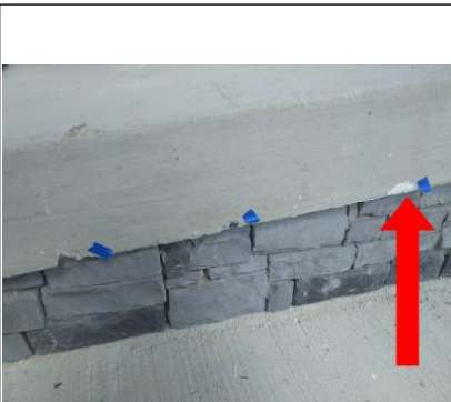
Chips out of bottom of the front porch, arrow points to paint spill.
