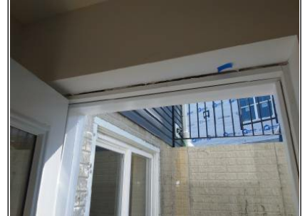
Dry wall not finished above egress door.
