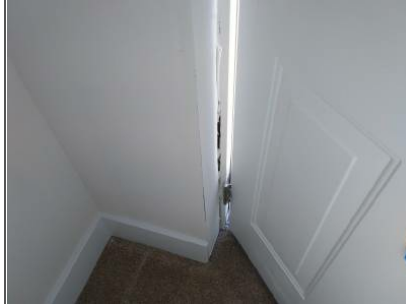
Drywall not finished behind egress door
