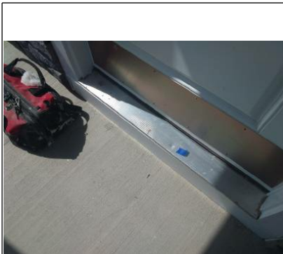
Front door threshold plate is dented and scratched.
