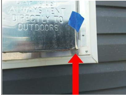
Bottom right corner of fireplace vent is dented.
