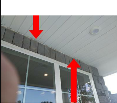
Mortar on the ceiling above the stone.
