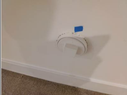
Rough finish around drain line clean out.
