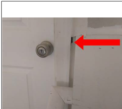
Gap between drywall and casing on the right side of the fire door.
