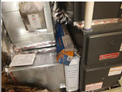
There is no backup filter left on the air handler.
