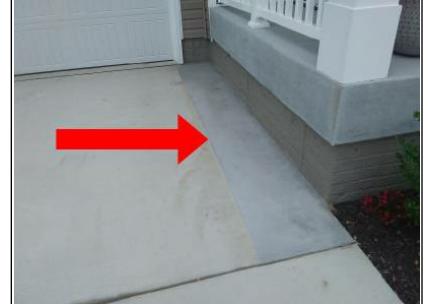
Finish on driveway surface at porch is inconsistent with the rest of the driveway.
