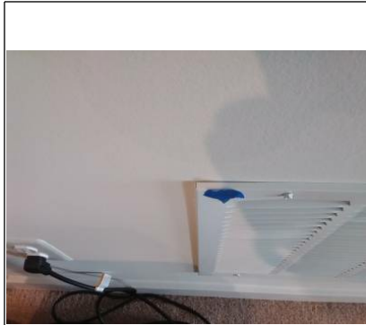
Return is not flush to the wall right of the utility room door.
