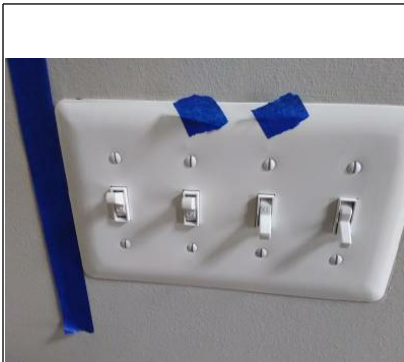
4 gang switch plate is overtightened creating dents. Switchplate is crooked.
