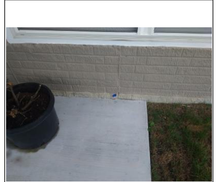
Foundation not painted above the patio surface.
