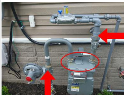
Gas meter supply lines are rusting.
