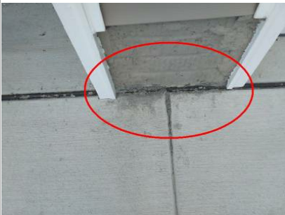
Concrete splatter on surface between garage doors.
