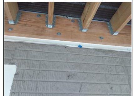
Paint over spray on flashing below the deck.
