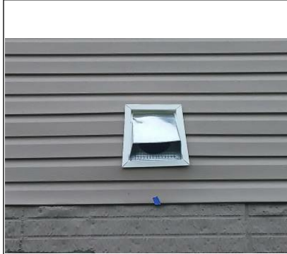
J channel not square around vent on the back side of the house.
