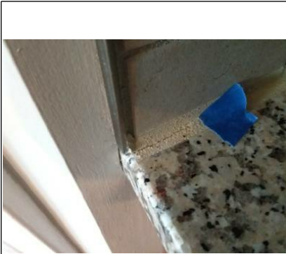
Grout crack between backsplash and counter to the left of the refrigerator.
