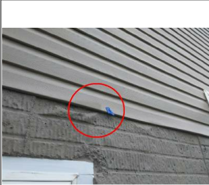
Paint over spray on siding on the back of the house.
