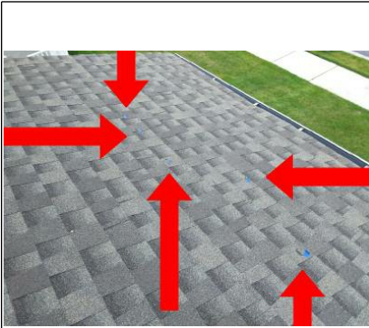
Surface of porch roof on the front of the house is damaged in several locations from ladder footings.
