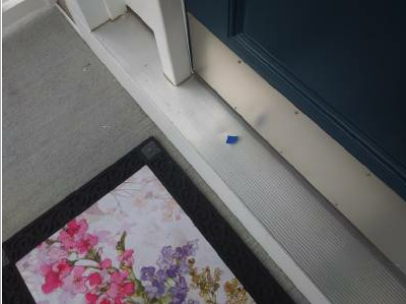
Front door threshold plate is dented.
