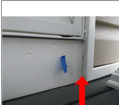
Threshold plate is loose and there is a gap between the threshold plate and the J channel on the right side of the sliding door.
