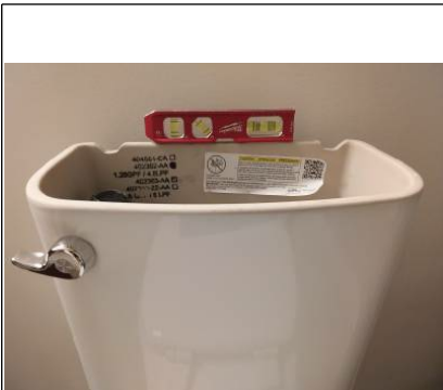
Toilet tank is not level, is pitched to the right.
