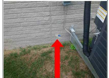
Paint missing on foundation to the left of the compressor.
