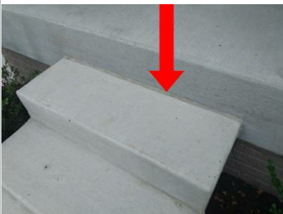
Expansion joint at top of steps inconsistent with the rest of the neighborhood. Ask builder for explanation of types of materials used.
