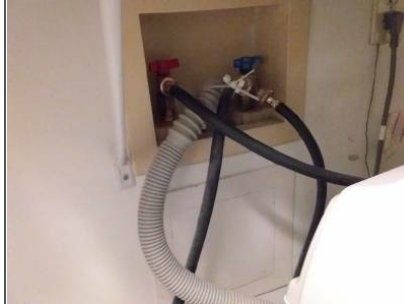
Recommend switching out water supply lines to reinforced supply lines. There are three supply lines.
