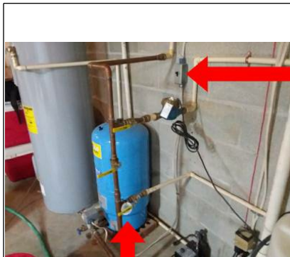
Water shutoff, switch for well pump
