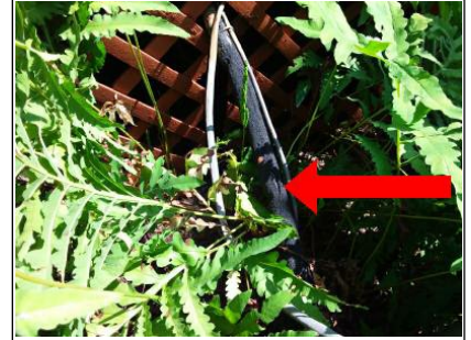
The insulation on the refrigerant lines should be replaced.
