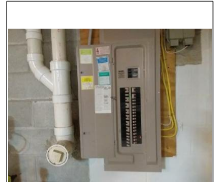
Panel is properly marked
