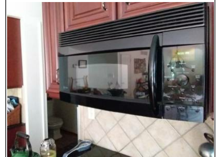
Microwave worked. Note that the fan recirculates air back into the kitchen.
