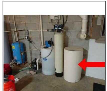
Water softener, salt reservoir
