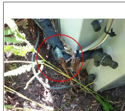
There is some torn insulation on the refrigerant line that should be replaced.
