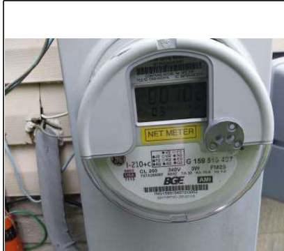
Electric service is 200 amps
