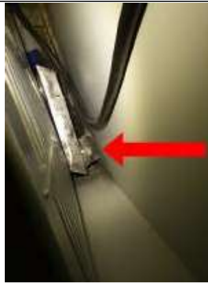
Ventline is loose at the connection and lint is collecting behind the dryer.
