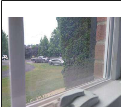
Top sash on left window appears to have an a broken seal
