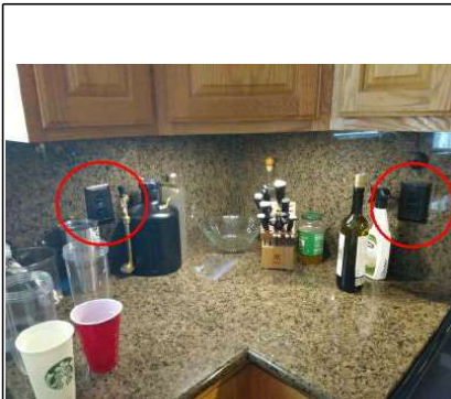
Two cover plates on the backsplash in the corner of the kitchen are loose.
