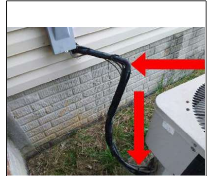
Insulation on refrigerant lines is damaged and should be replaced.
