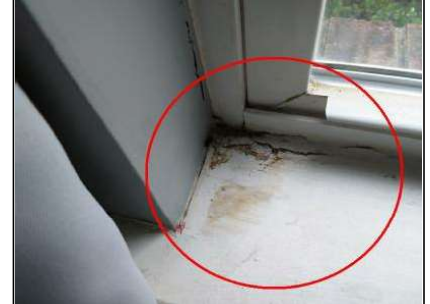
Signs of water damage on the windowsill.
