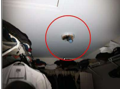
Globe for the light fixture in the closet is missing
